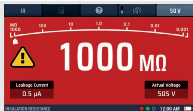
Fig 21: Insulation test in progress
